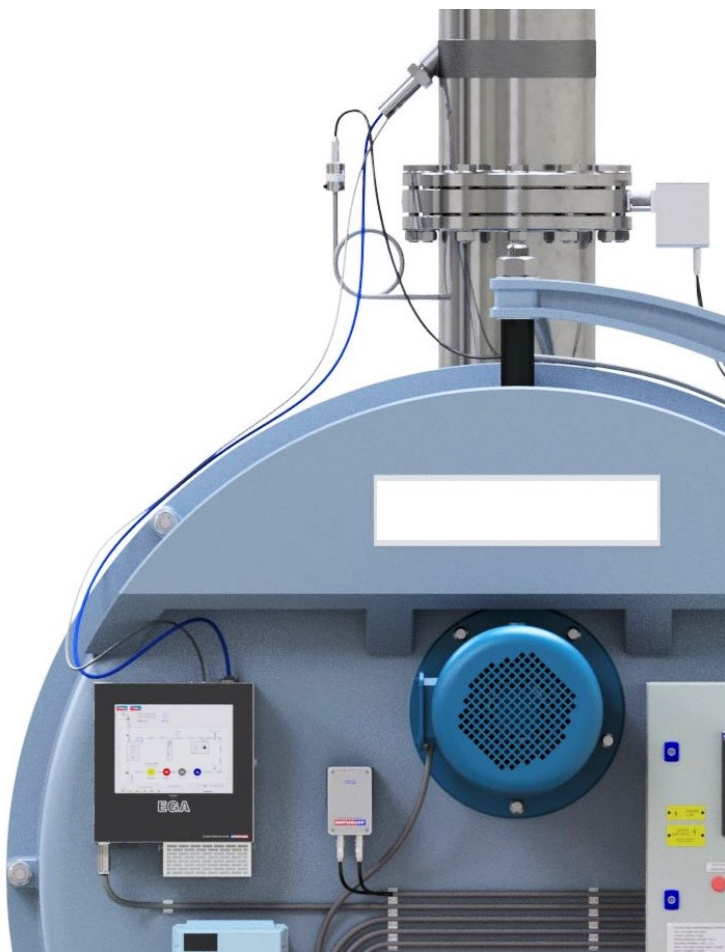
Figure 1.6.4.ii Incorrect installation of the sampling probe: a gully is formed in the sampling line will cause blockage
