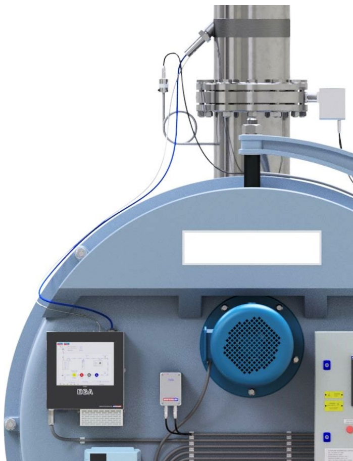
Figure 1.6.4.iii Correct installation of the sampling probe: the sample can flow down the sampling line with no restriction.
